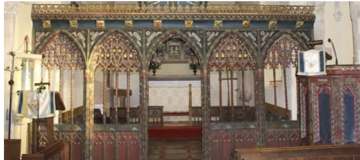
The carved oak chancel screen , of 5 bays dates from the mid to late 15 th century, perpendicular tracery, cusping, little shields and early stenciling. Further additions and improvements were made to the Church during the time of Sir Nicholas Wadham, who succeeded to the Manor of Rewe in 1495.
