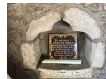
An excellent trefoil headed piscina remains on the S side of the chancel with a drain used for washing communion vessels. Note how rough and crooked are the stones that have been used in the masonry round it. A tile commemorates the lives of Thomas & Susannah Cole.
