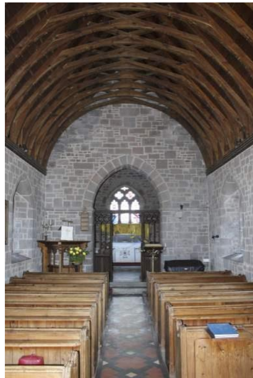
ROOF – pitch-pine roof; arched principals & purlins in the Chancel, Trussed rafters in the Nave
