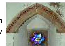
Ogee Arch and Window
