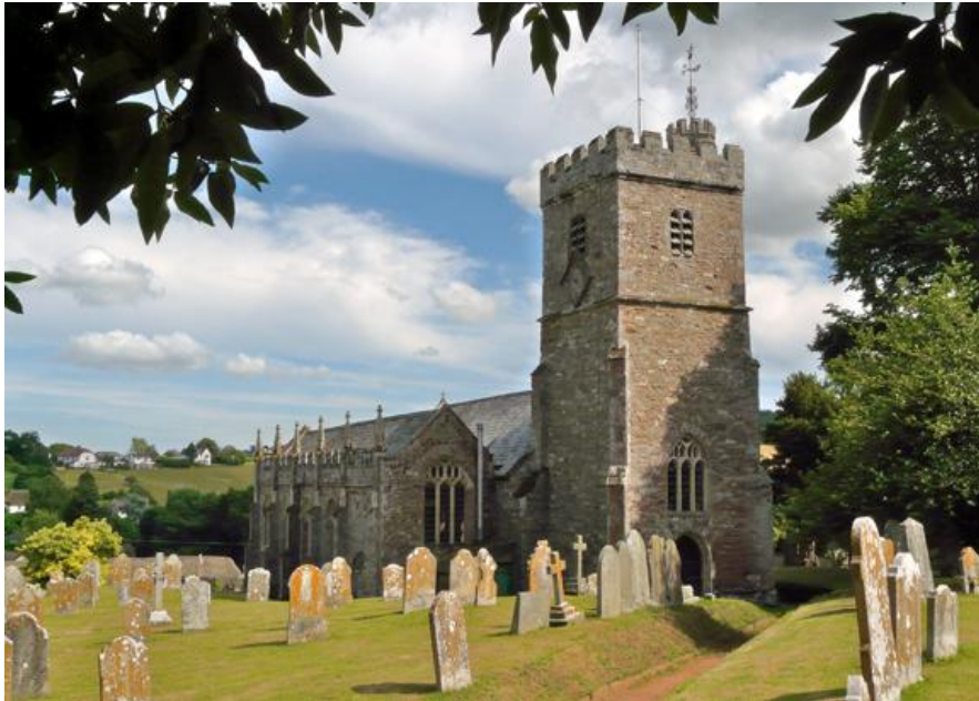
The northern side of the Church and older part of the Church yard. Each of the buttresses on this side is topped with a pinnacle.
