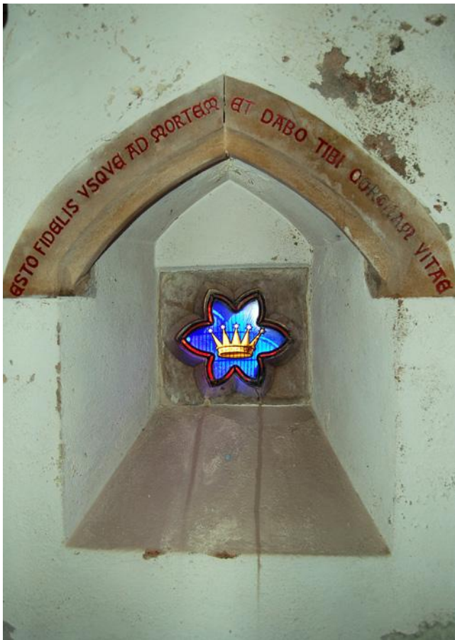
The painted Ogee arch in the south aisle
